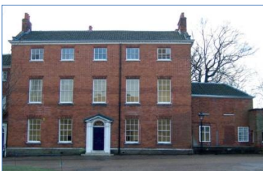
M+A Partners head office, located within Norwich Cathedral Close.
